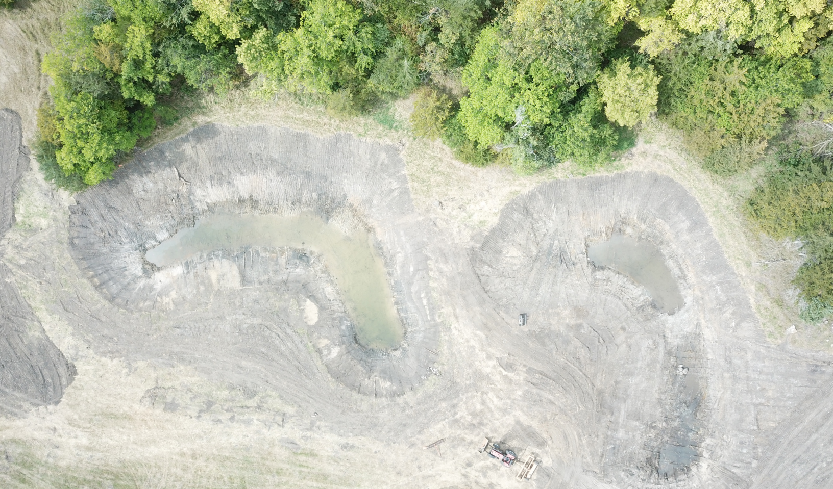
Drone photo of restorations immediately after completion. © City of Webster City
