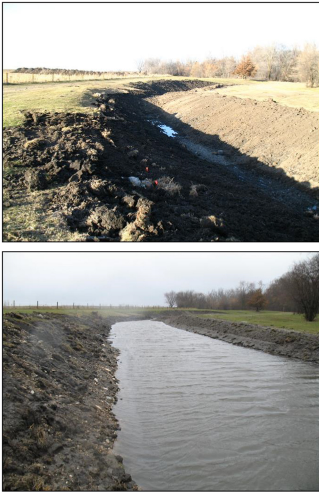
Fig. 2. Photographs showing oxbow excavation (top) and oxbow filled with water (bottom).
