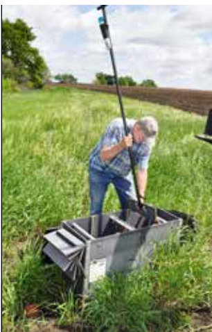
Conservationist Bruce Voigts inserts a panel into a water-control structure that intercepts field tile water and backs at least some of that water into a perforated tile within a grass and tree buffer along a stream in north-central Iowa. The perforated, underground tile releases the water into the buffer's soils, where roots of the grasses and trees filter and remove nitrates from the water.
