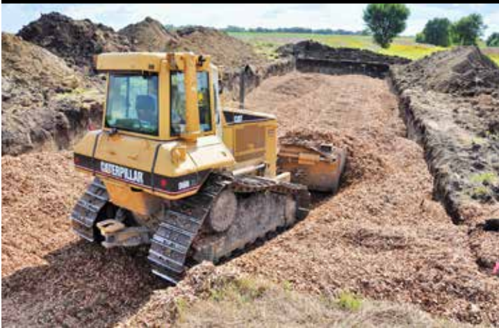
A bioreactor intercepts tile water and runs it through a bed of underground wood chips before it reaches a stream and leaves the farm.
